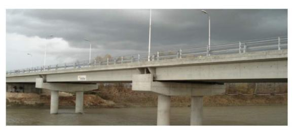
New bridge has a total length of 90 m and it consist of 3 spans.
